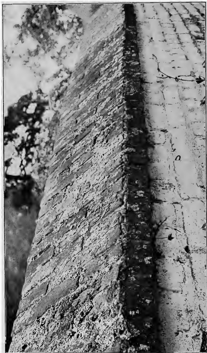
A SECTION OF THE LICHEN-COVERED GARDEN WALL
